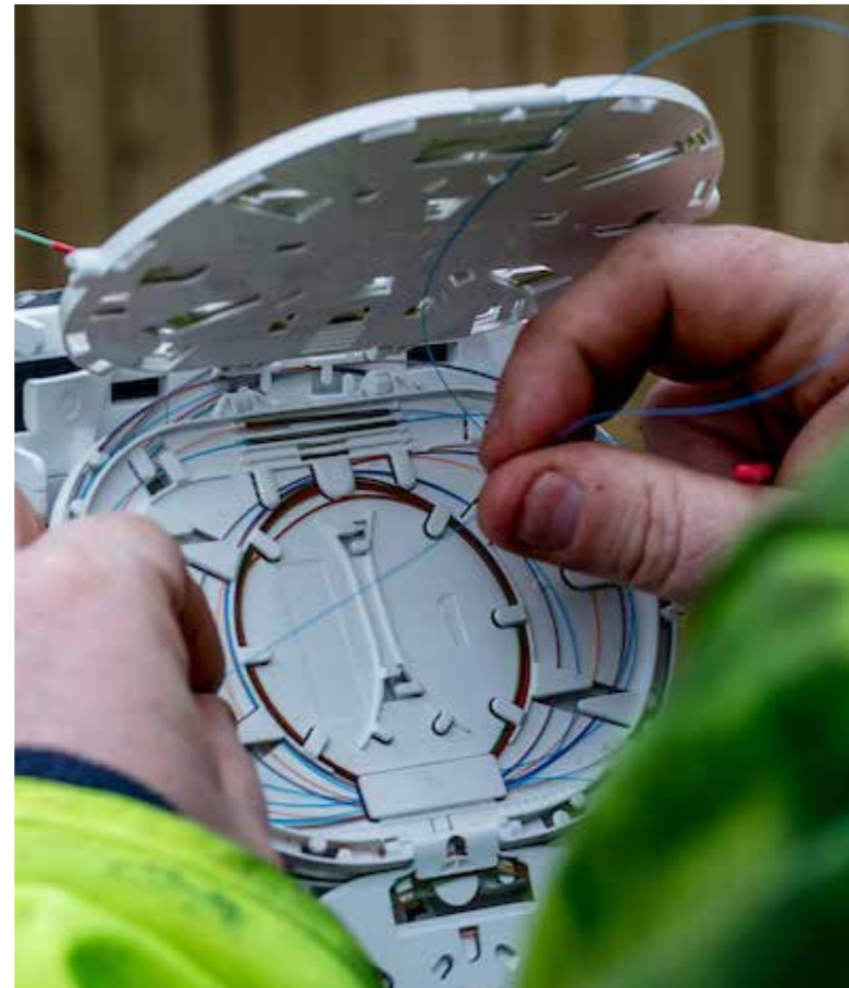
Engineer Graham Wray carries out fibre splicing and testing, simply put, fibre optic splicing involves joining two fibre optic cables together.
